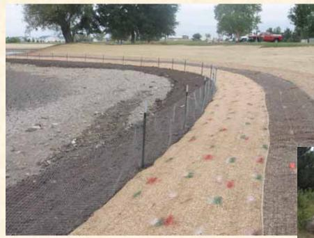
Observed Normal Water Level Surveyed and Flagged to Mark Centerline of TRM
